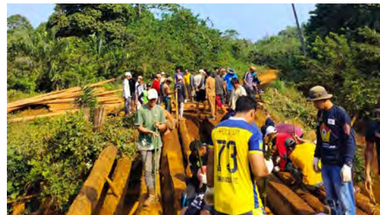
Perbaikan Jembatan Desa Tambakua Bridge renovation at Tambakua Village
